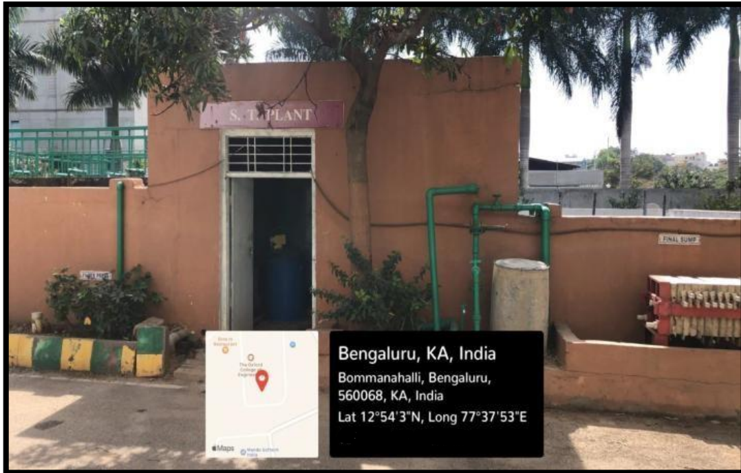
Sewage Treatment Plant
